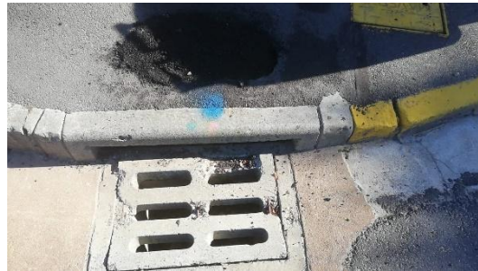
Repair hole in pavement C/O Washington Street and 11 Avenue
