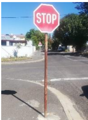
Repair rusted stop street pole, C/O Washington Street and 8 Avenue
